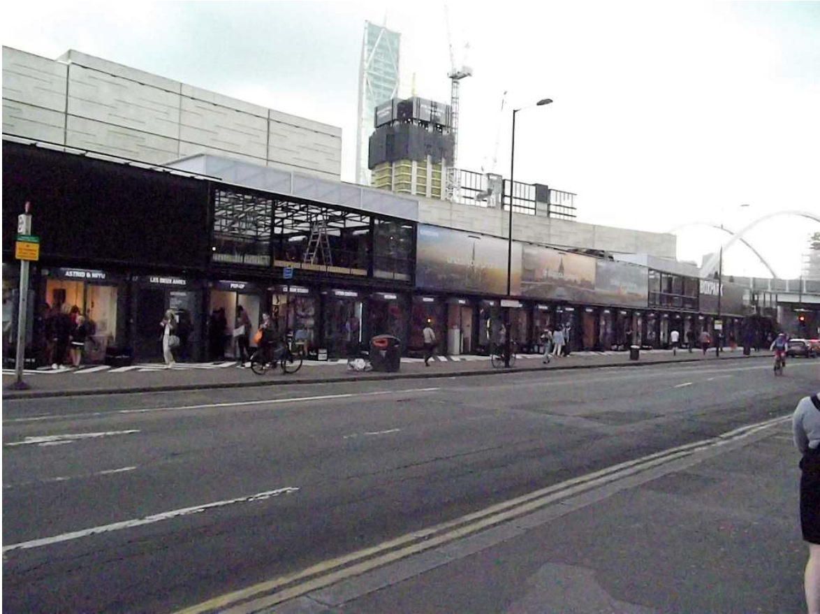
Figure 3: BOXPARK site from end of Ebor Street
