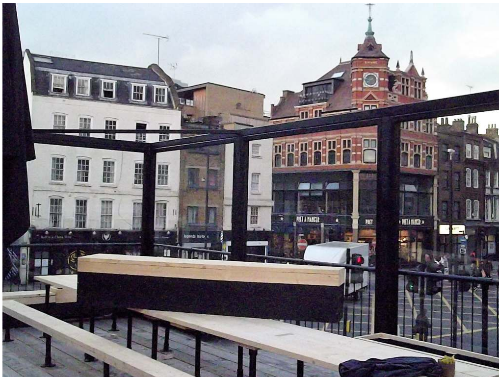
Figure 7: End terraces now enclosed with glass walls which form a significant acoustic barrier
